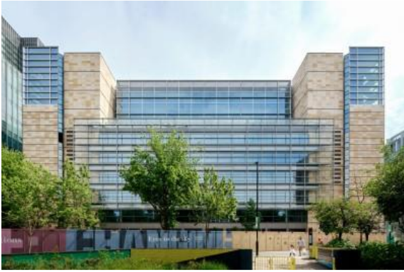
1 Triton Square, London British Land 3000 m 2 of remanufactured glass facade
