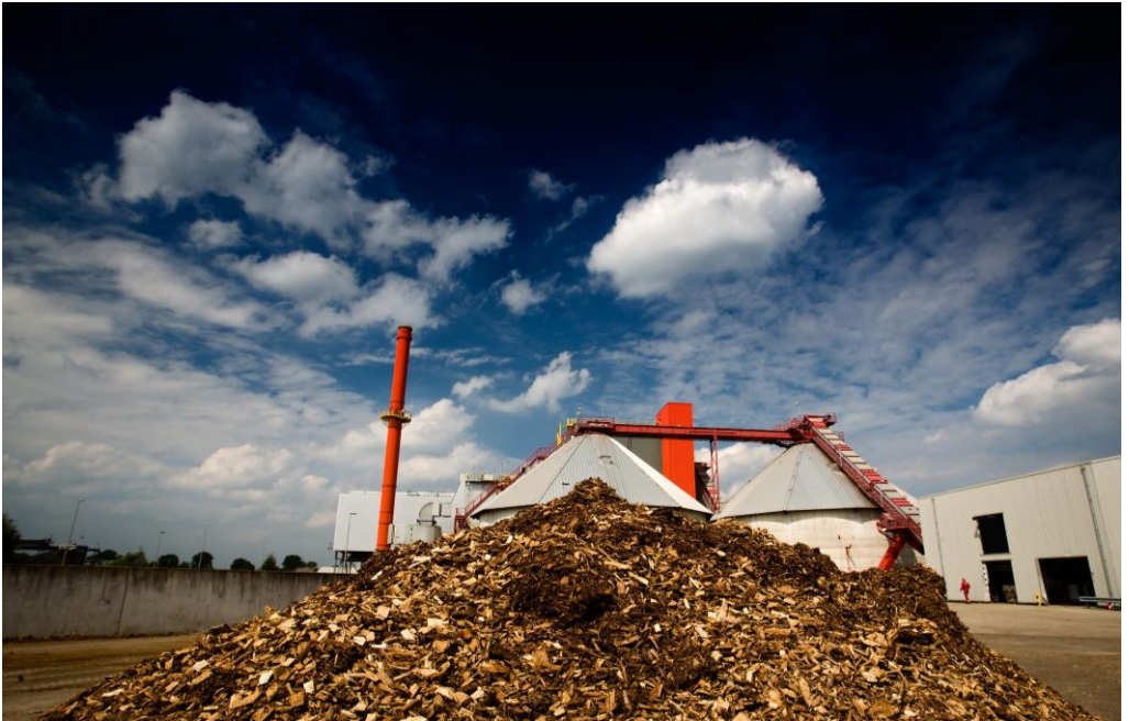
Bio-energy plant in Cuijk
